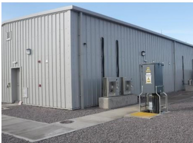
Image 4: AIS control building (source - RWE)
